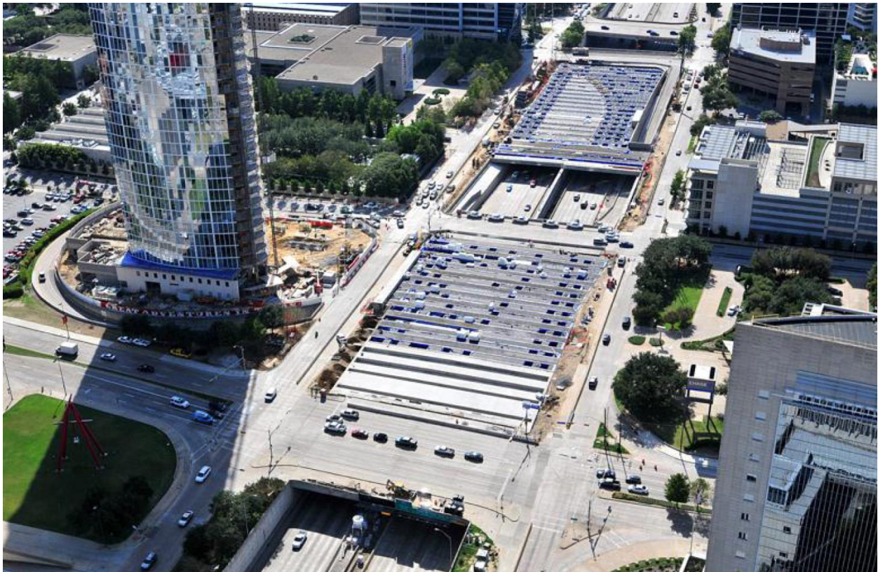
Figure 24 - Construction of Klyde Warren Park's structure. The dark rectangular holes are where trees were planted. 105
